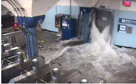
FIGURE 4: NYC Subway Flooding (Hurricane Sandy)
